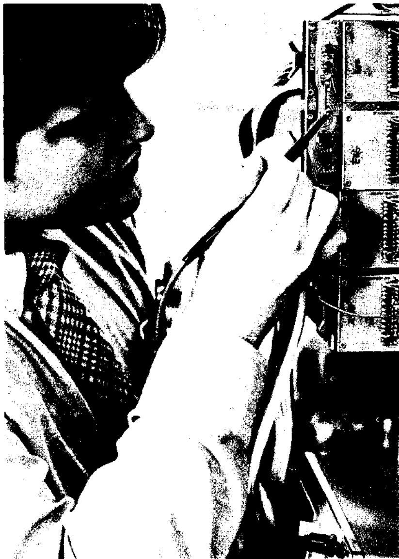
DEC engineer checks out part of a K Series control system.
