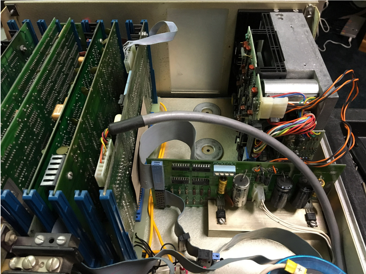
Internal rear view showing the buffer board.
